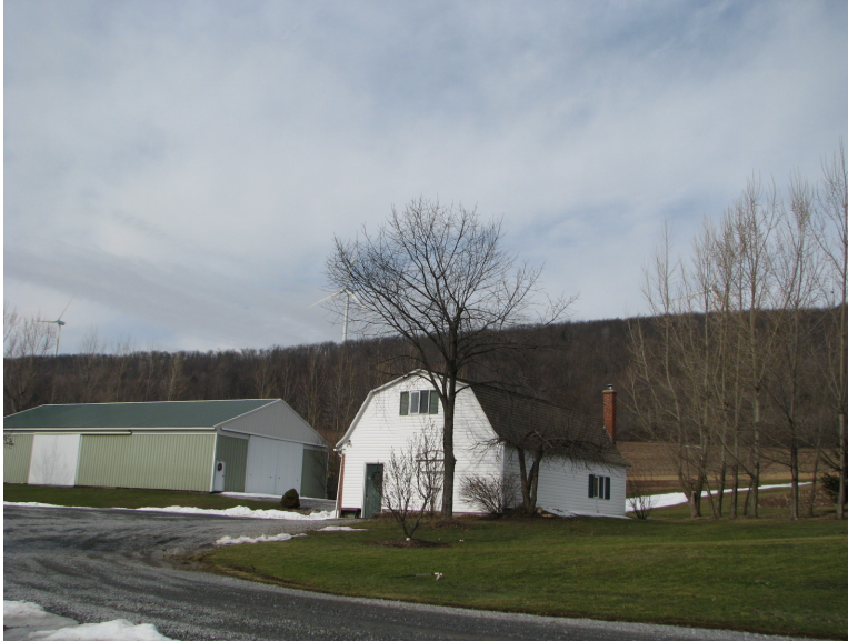
Figure 8: View from the Stull Monitor Looking North towards Turbine A20
